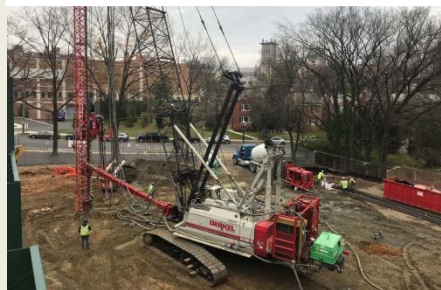
Drilling in Progress
