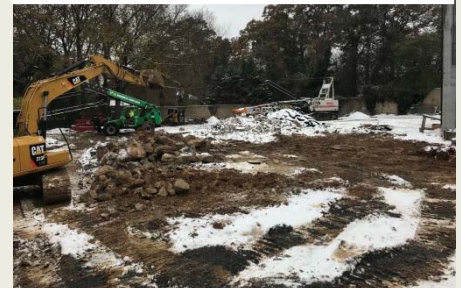
Asphalt & Concrete removal
